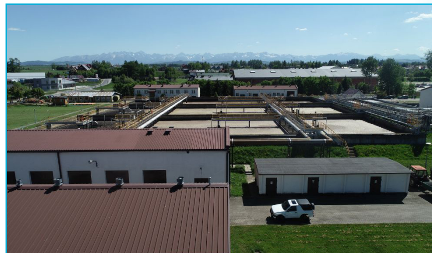
Photo 8. Sewage treatment plant. Source: Nowy Targ City Hall
