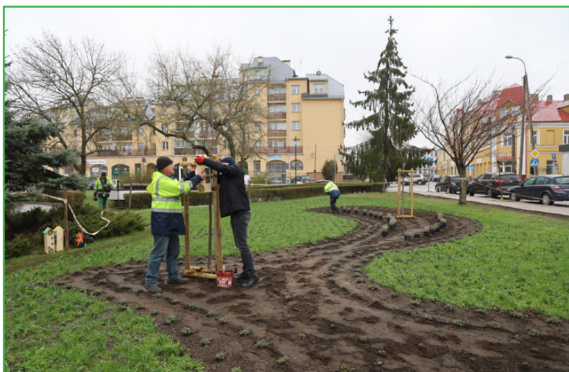
Photo 64. "Butterfly corner" in progress. Source: Ostrów Mazowiecka Town Hall
