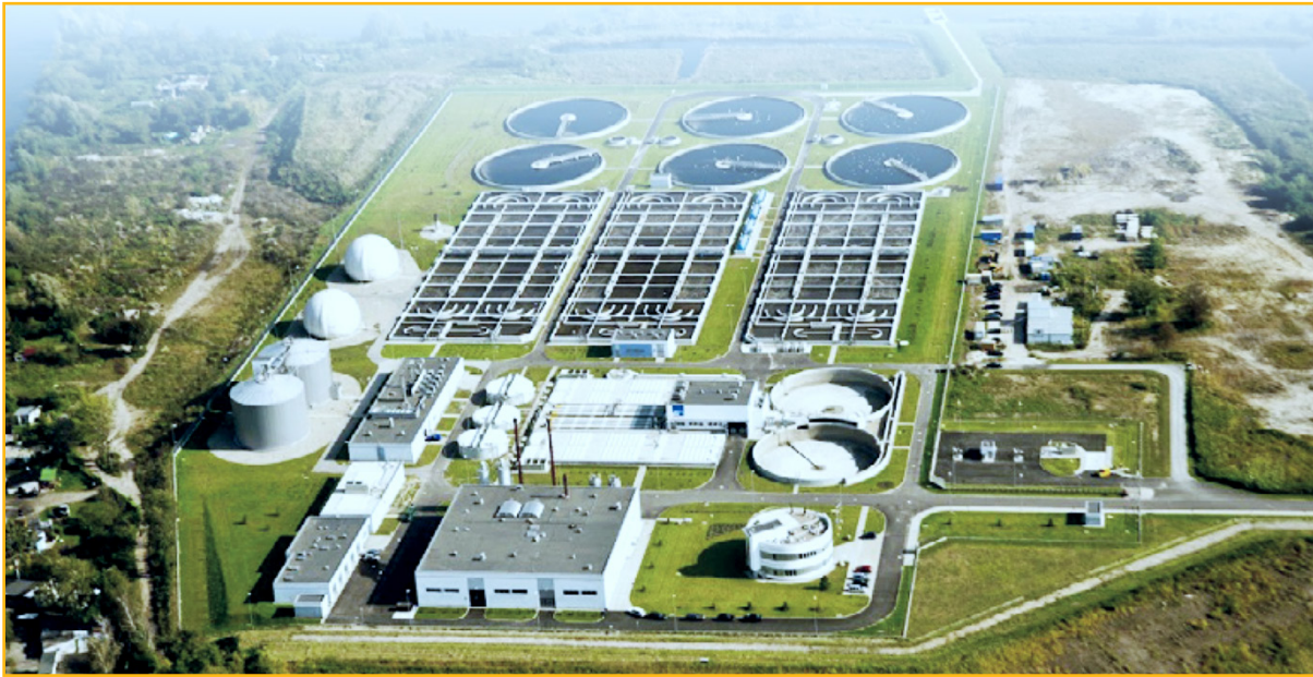
Photo 12. Sludge fermentation chambers and gas tanks of the Pomorzany sewage treatment plant in Szczecin Source: Water and Sewerage Company in Szczecin
