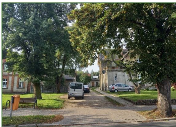
Photo 45. Ulica Mickiewicza 32 - state before the project implementation. Source: Town Hall in Śrem
