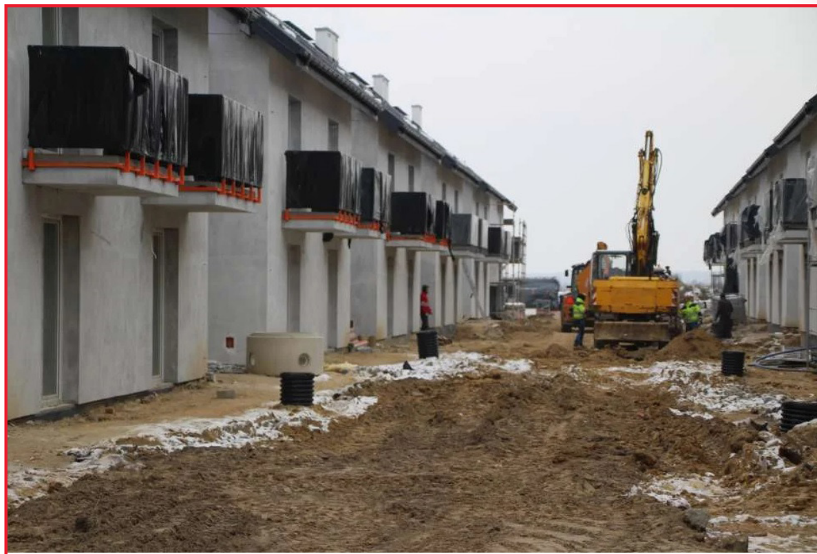
Photo 1. Construction of Apartments Plus in Potarzyca. Source: Town Hall Jarocin
